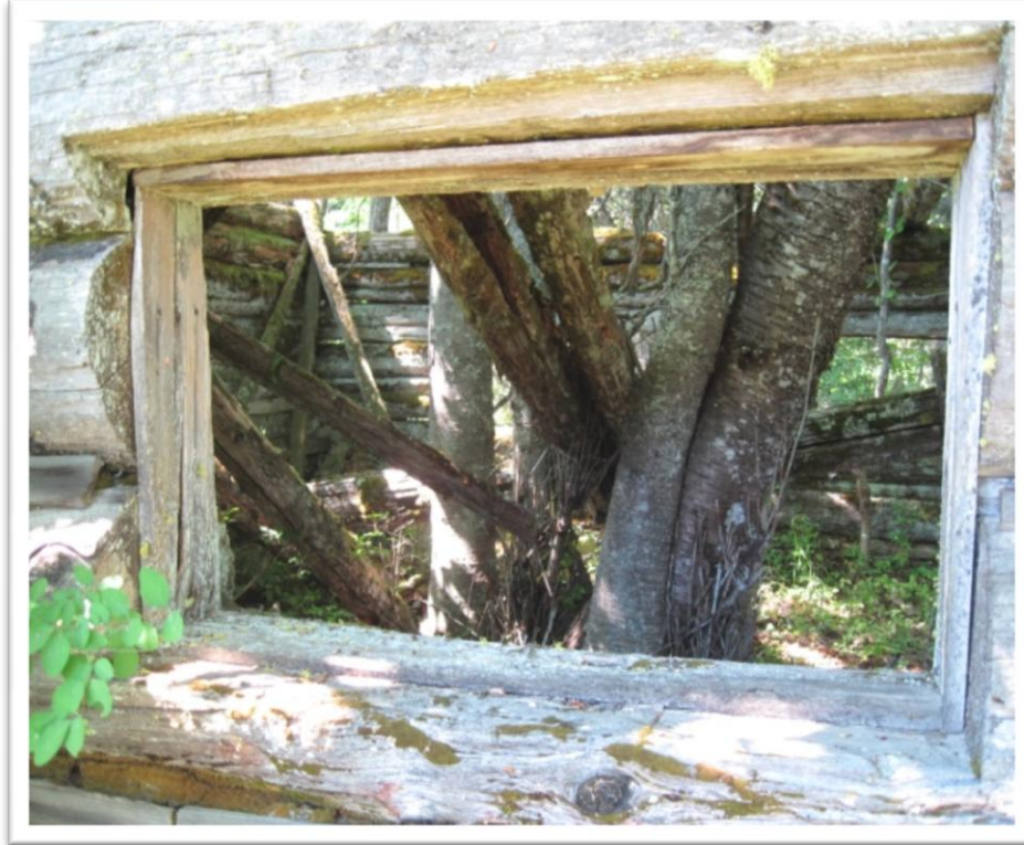
Figure 5. View into the structure with a tree growing from within.
