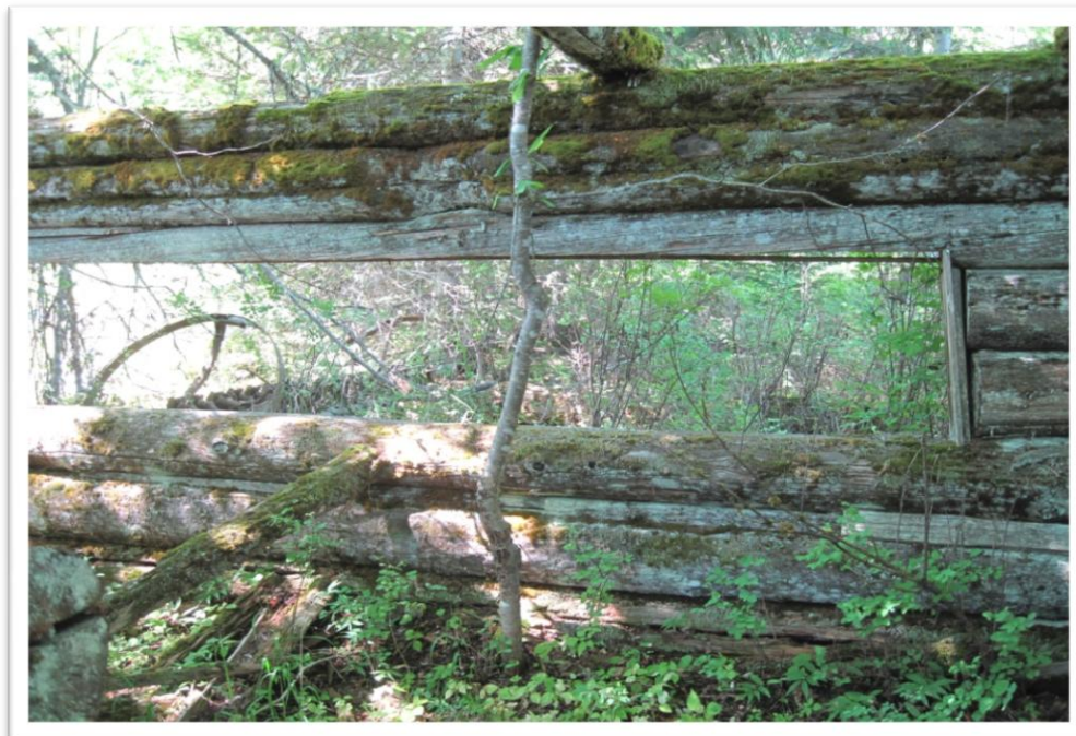
Figure 4. View out of the structure through a particularly long window.
