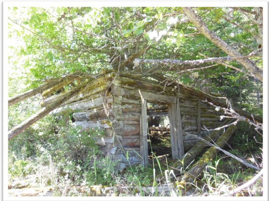
Figure 2. View of structure with fallen tree on roof.
