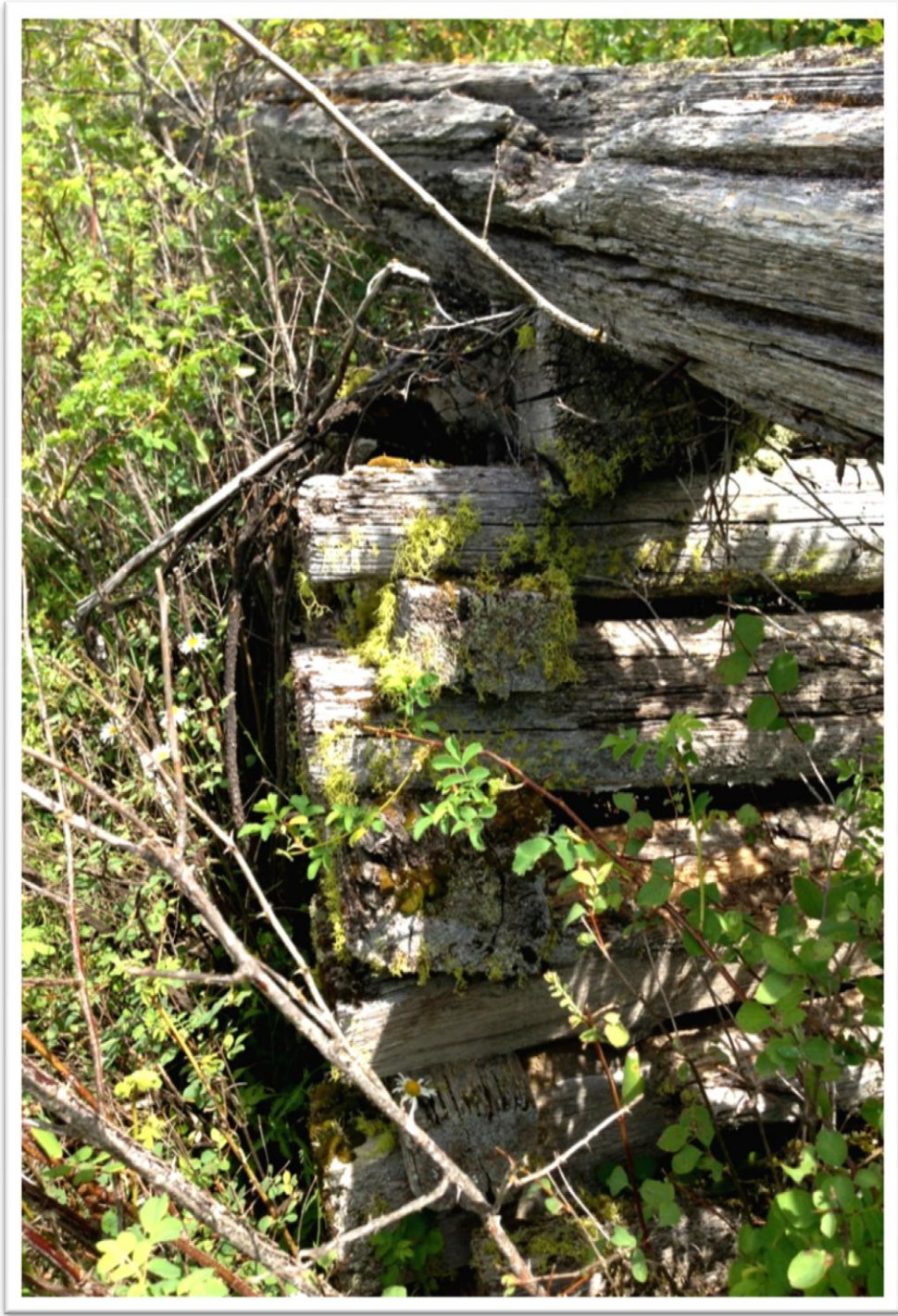
Figure 2. Corner notching on remaining portion of structure.
