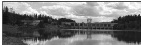
Downstream side of Albeni Falls Dam with powerhouse on left and spillway on right
